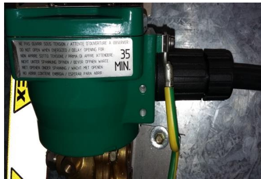
Figure 7: Cable system with direct entry
