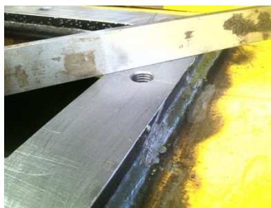
Figure 9: Checking flange faces with a straight edge
