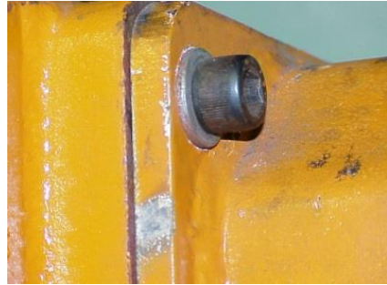
Figure 3: External flange joints
